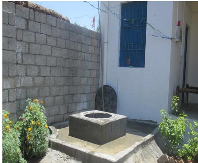
Figure 6: A rehabilitated well
